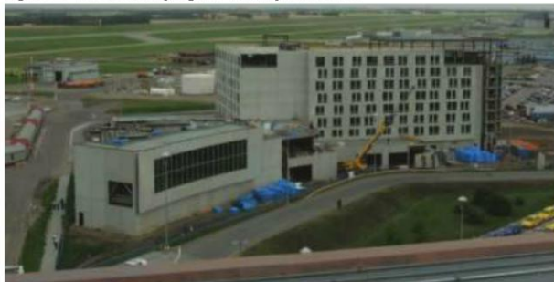
Figure 2: Construction progress in early June 2012
