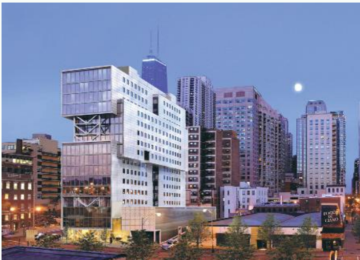
Rendering of Chicago Staybridge Suites hotel staggered truss project scheduled for completion in 2009, left. Typical 3-D model of standard staggered trusses supporting hollow core slabs. Rendering: Valerio Dewalt Train
