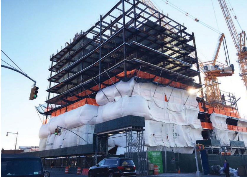
◀ Construction of the 11-story office tower.
