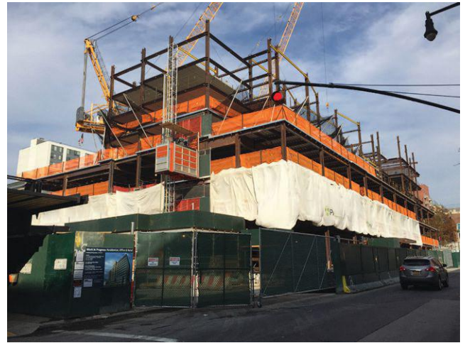
▲ Construction of the residential building.
