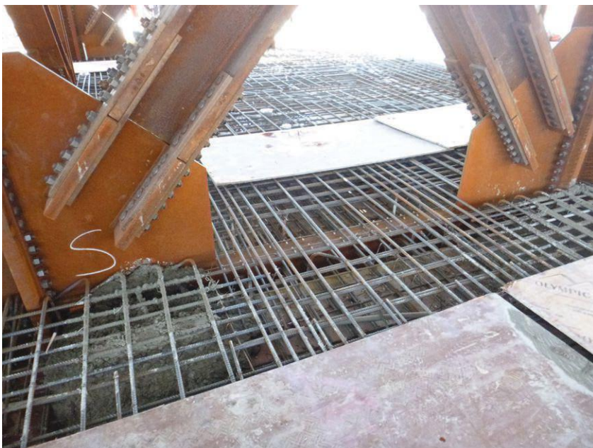
▲ A strap beam erected on-site.
