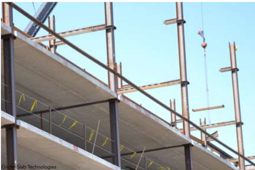
▲ Figure 5: Tree columns in place.
