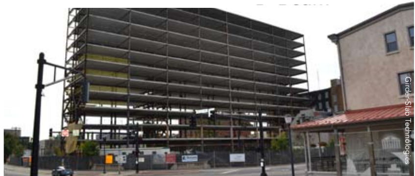
▲ Figure 2: The fully erected and planked structure in mid-September 2011.
